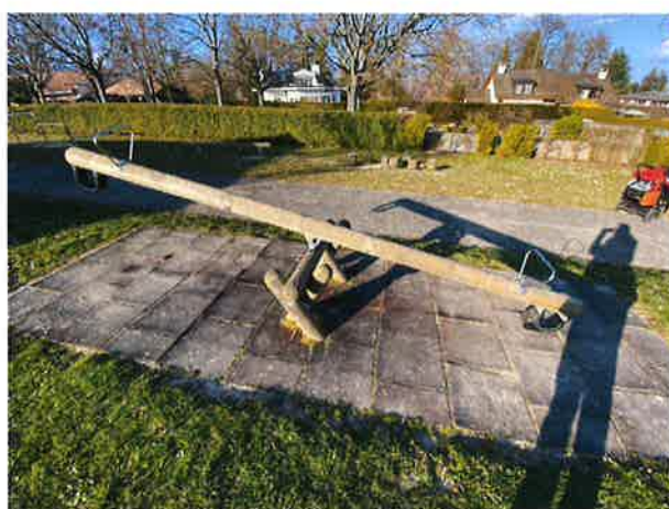
Etat du sol souple, joints apparents, etc ...
